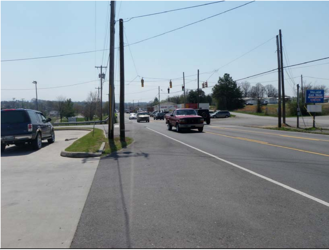
Photo 3: South view of Defoe Circle intersection from approx. Sta. 109+00 on SR-33.
