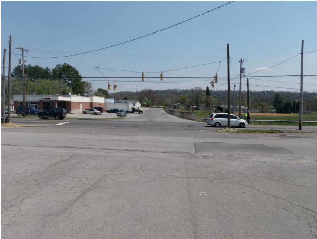
Photo 2. East view of SR-33 intersection from carwash parking lot.
